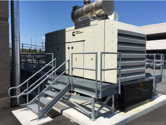
Generator Combo Unit
