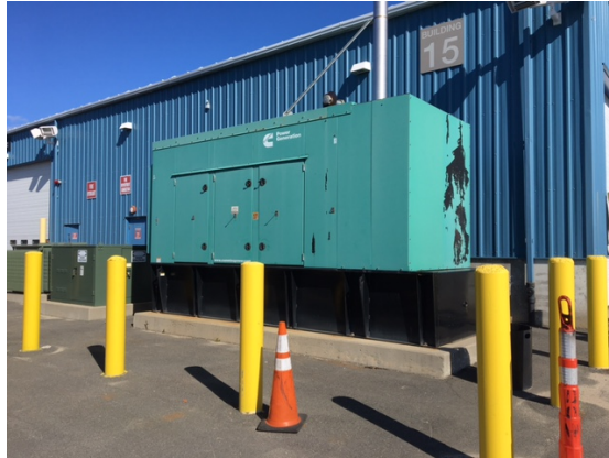
Elevated Platform at CTDFC
