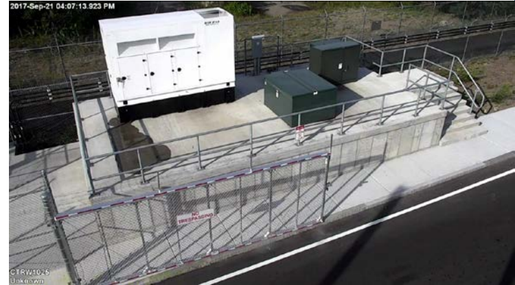
State Police Generator
